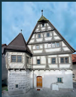
Imitation of hewn stones painted on the plastering of the Little Big House
