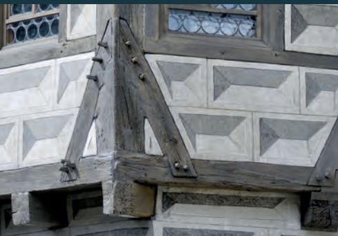
Imitation of hewn stones painted on the plastering of the Little Big House
